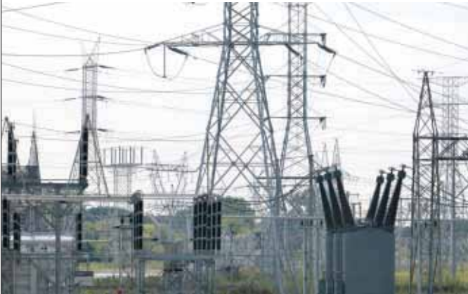
Transmission Line & Tower-erection projects
