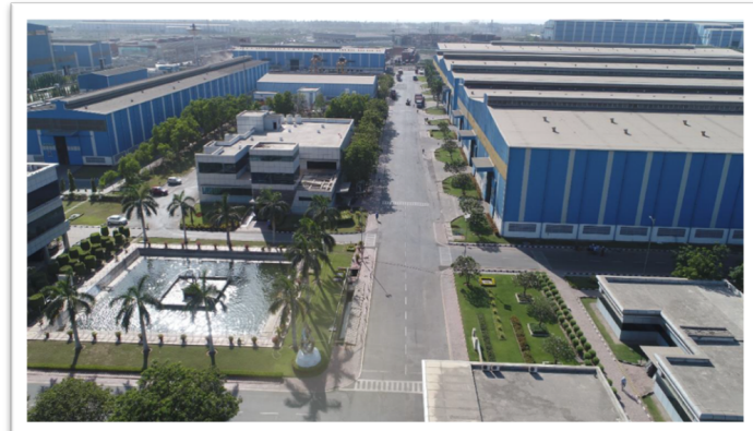
L&T MHI Power Boilers Pvt. Ltd. – Hazira, Surat – Manufacturing Facility
