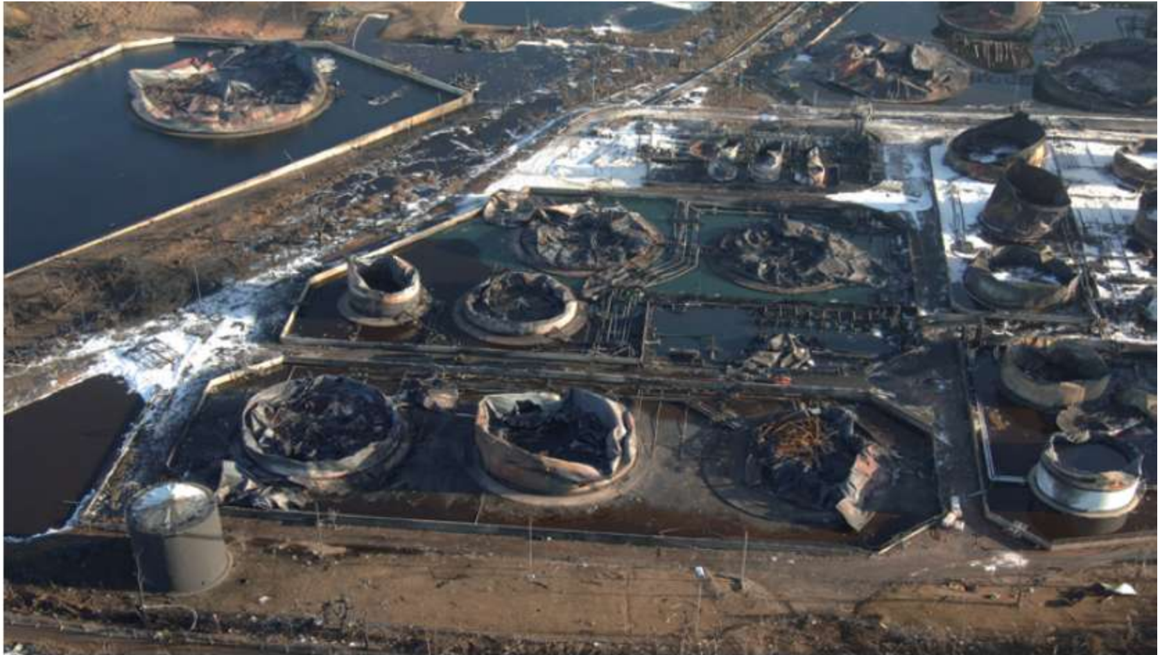
Figure 6 Buncefield after the incident: Tank 912 is in the centre foreground and Tank 12 is in the top left of the picture © Chiltern Air Support
