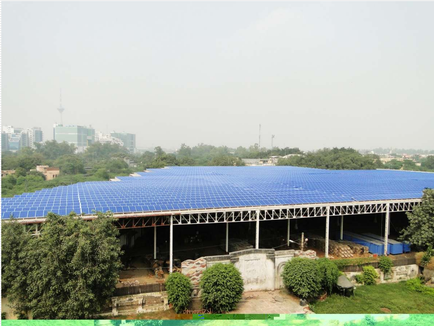
1 MW PV (Crystalline Silicon) Grid Power Plant at New Delhi (Solar RPO arrangement)
