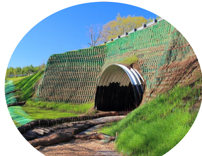
Reinforced Soil Walls
