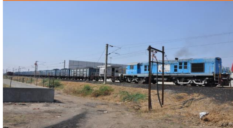
Dahej - Bharuch Railway line
