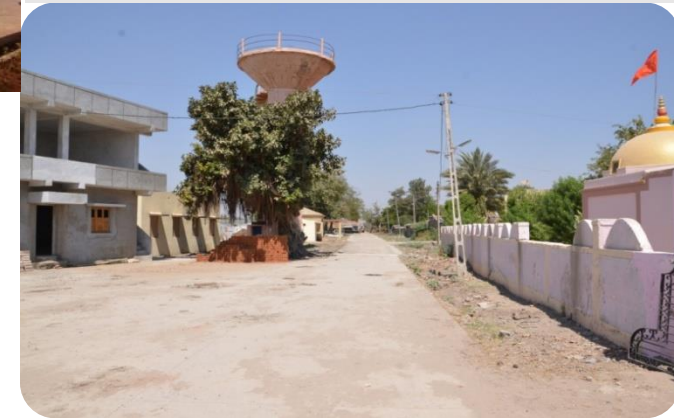
Potable Water Supply Scheme - Rs 2 crore
