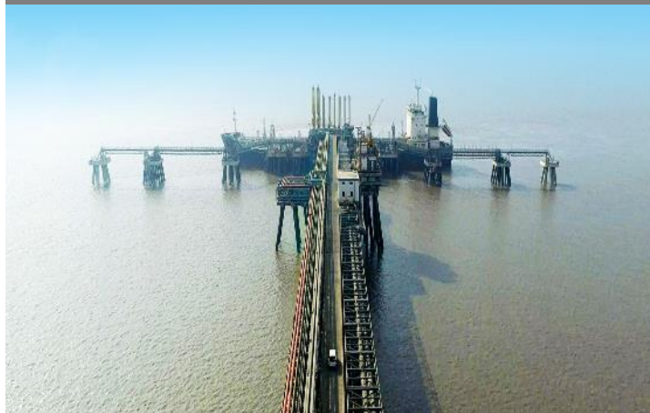
GCPTCL (Liquid Chemical Terminal)
