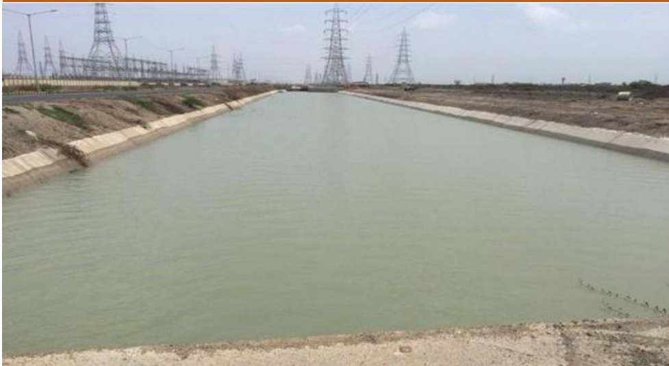
Raw Water Reservoir
