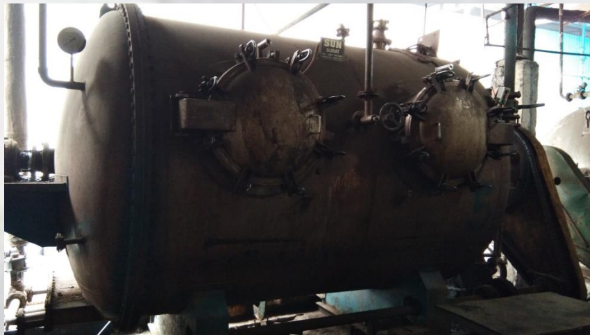
Drum Machine at T.M. Patel with PLC
