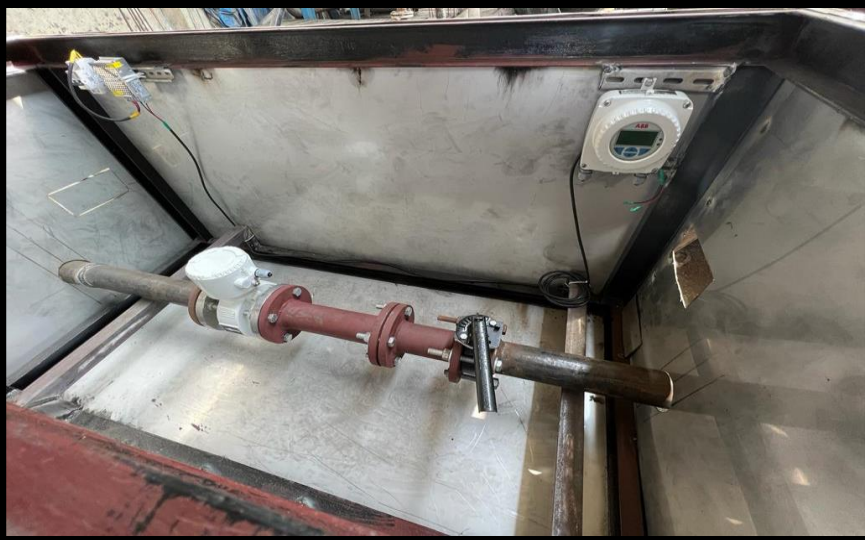
FLOW METERING SYSTEM FOR RO PERMEATE AT MEMBER INDUSTRY
