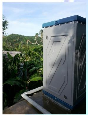
At Mantaray Island Resort in Fiji, a BioGill system is treating 14,000 litres of wastewater each day from the kitchen, laundry, showers and composting toilets.
